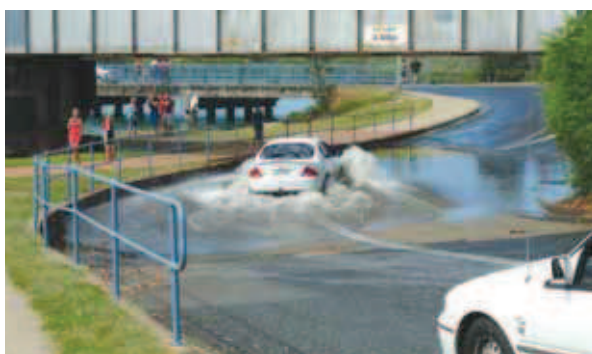
Coffs Creek penetrating back up stormwater system, 12 Jan 2009 king tide – Mel Bradbury
